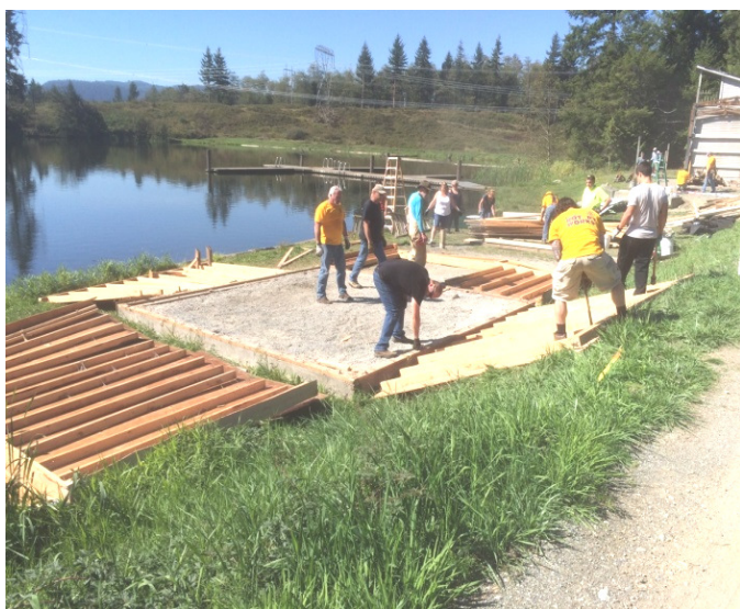
Arlington Rotary demolishing the old beach structures
